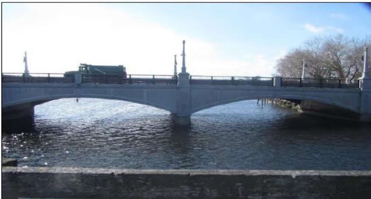
Photo No. 7: Looking Downstream From Top of Bridge (2019 Photo)
