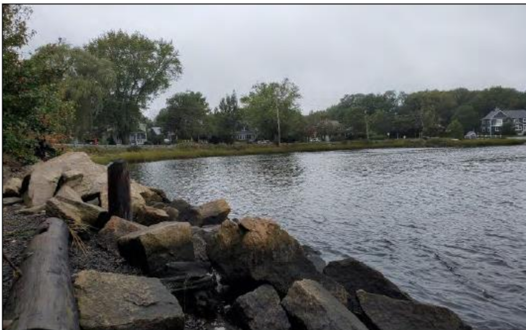
Photo No. 12: North embankment at east abutment looking east
