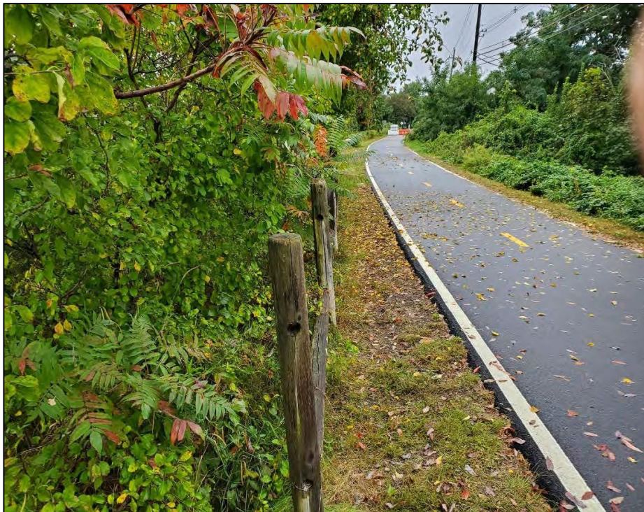
Photo No. 3: West Approach Looking West
