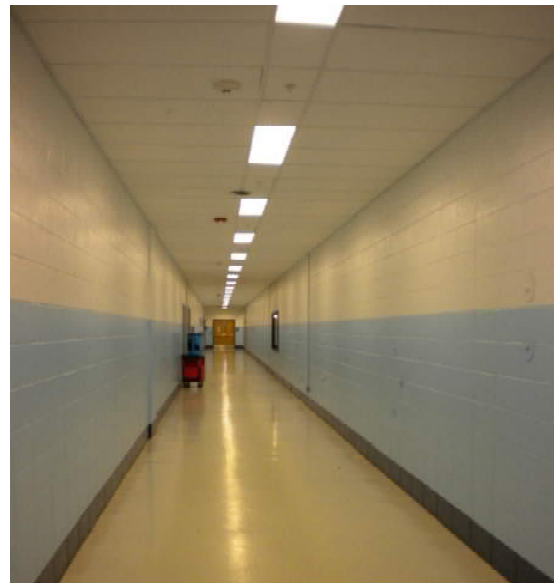
Photo C2: Existing West Corridor
