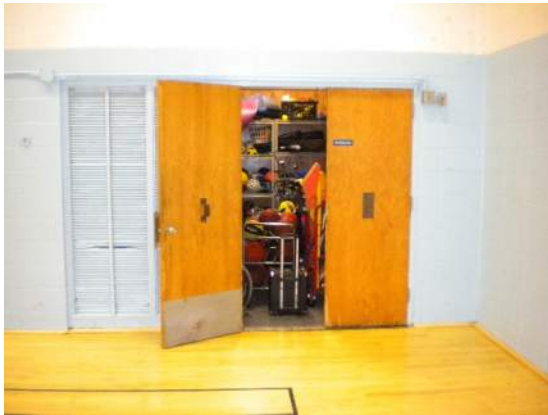
Photo B5: Existing Doors and louvers.
