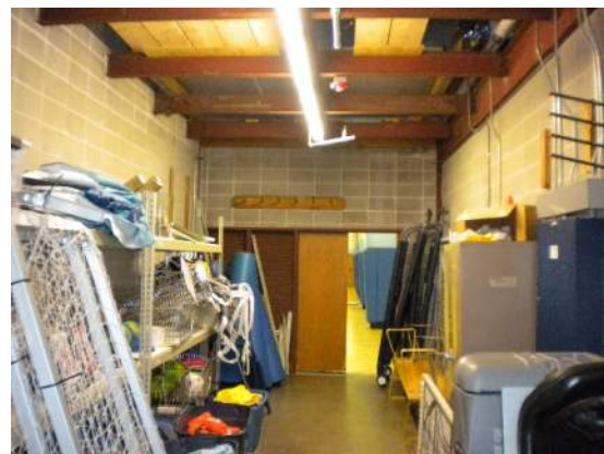
Photo B4: Existing Storage Room.
