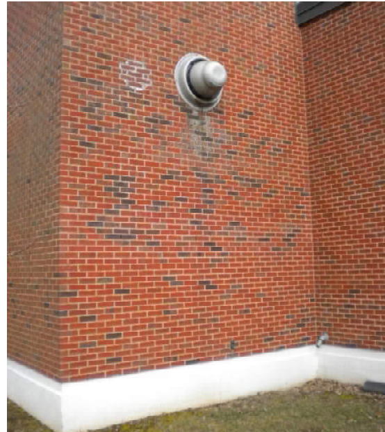
Photo A16: Mortar patch.
