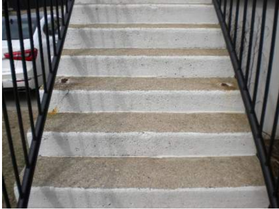
Photo A7: Existing railing sleeves.
