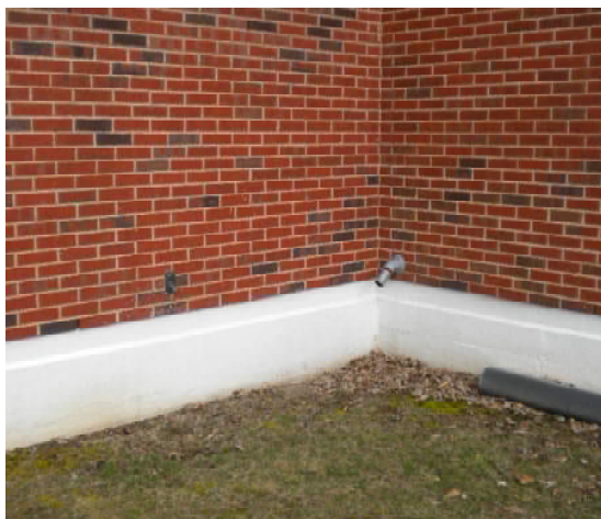
Photo D3: existing pipe penetration/hose bib
