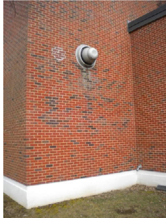
Photo D2: Laundry Room Exhaust.
