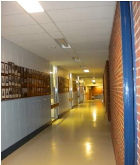
Photo C11: Existing South Corridor
