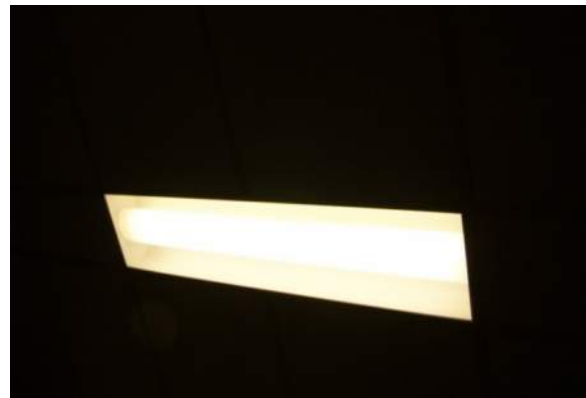
Photo B1: Lighting in corridors.
