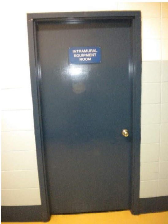
Photo B7: Existing door to corridor.
