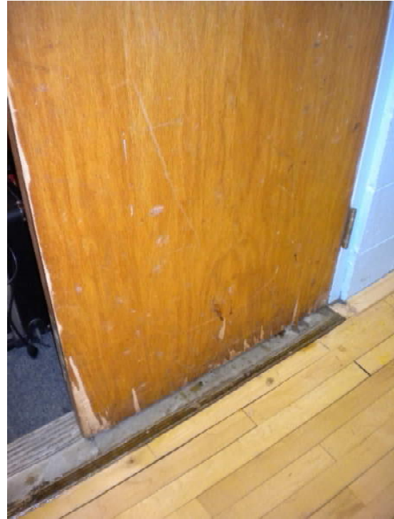
Photo B6: Existing Wood door.
