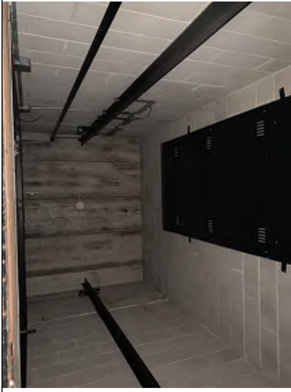
Top of Elevator Hoistway.
