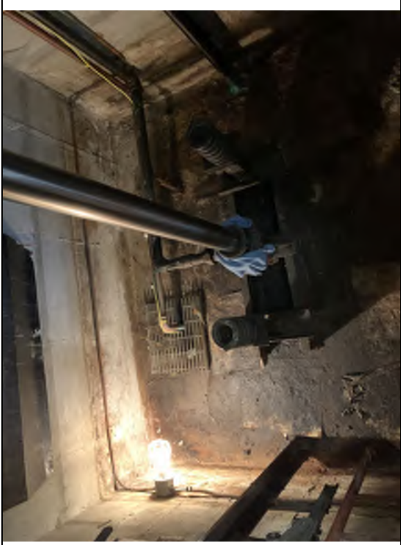
Elevator Pit Area
