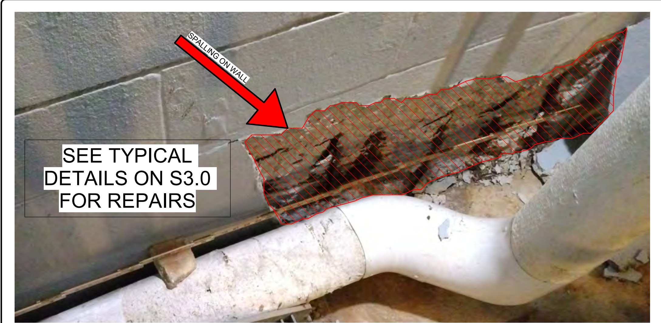
A1 PHOTOGRAPH OF DEFICIENCY - DETERIORATED FACE OF CONC. WALL A DEFICIENCY A - FIRST FLOOR WALL SPALLING NO SCALE
