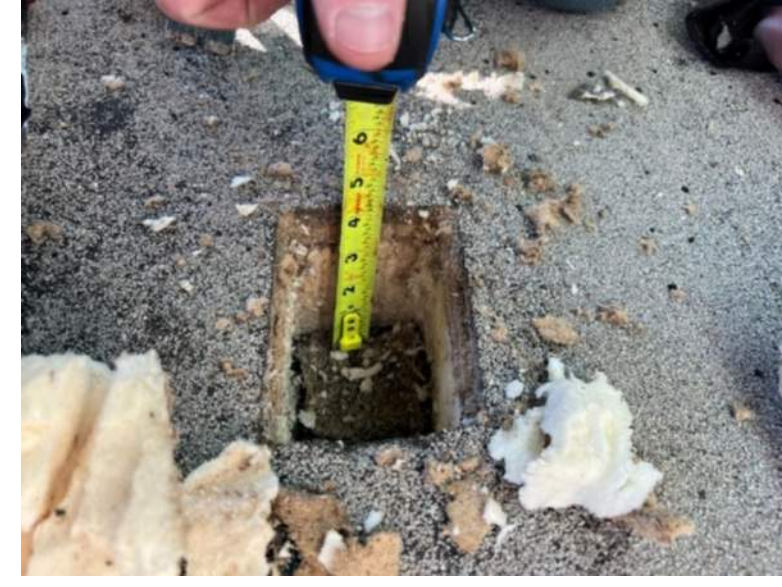
① UPPER ROOF TEST CUT 1/2" = 1'-0"
