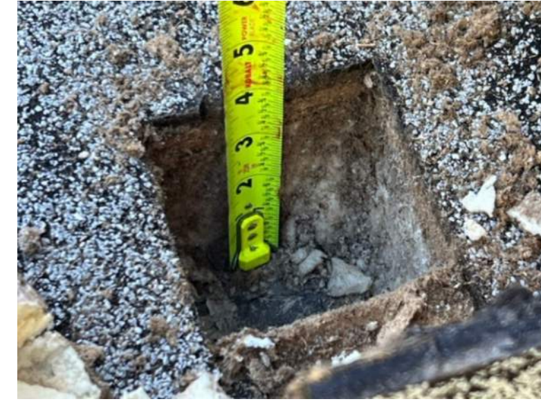
② LOWER ROOF TEST CUT 1/2" = 1'-0"
