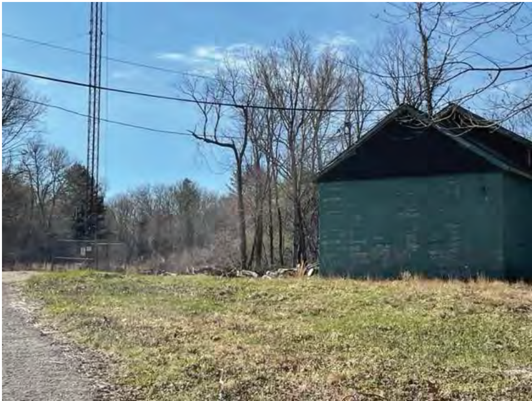
Photo 3 – URI Radio Tower Control Room
