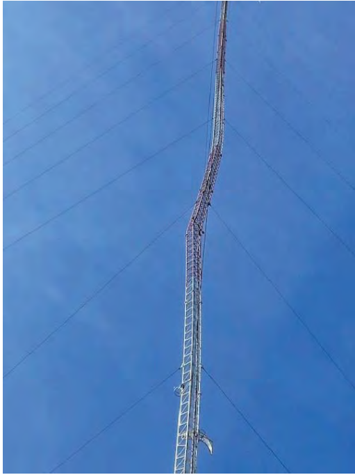
Photo 1 – URI Radio Tower to be demolished
