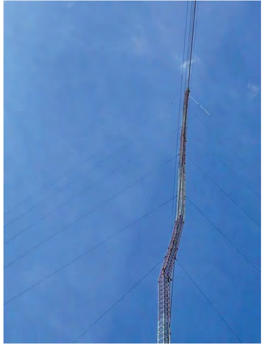
Photo 2 – URI Radio Tower to be demolished
