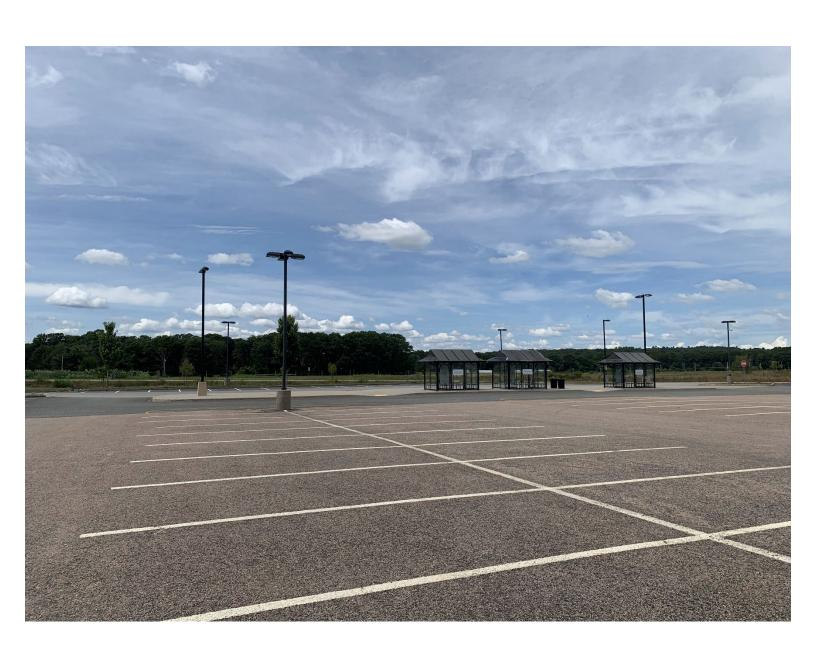
This feature is a Pervious Asphalt Parking Lot containing 408 parking spaces. This is a commuter parking lot. It contains a central located bus shelter and has solar roof canopies.
