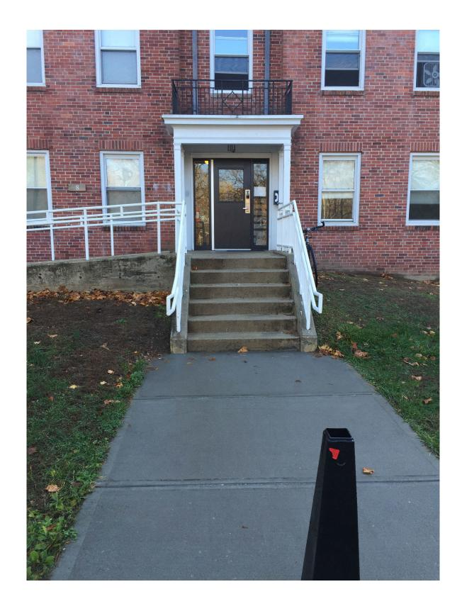
This feature contains a Concrete Ramp. There are Ramps/Walkways 4 feet wide and approximately | Total Area: 120 square feet. 30 feet total length.
