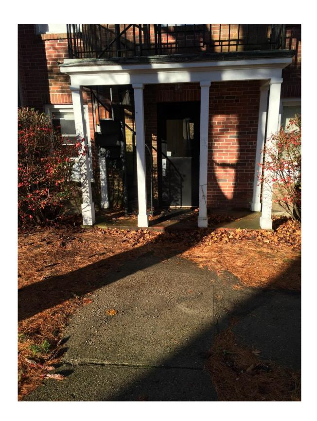
This feature contains a Concrete Ramp. There are Ramps/Walkways 5 feet wide and approximately | Total Area: 150 square feet. 30 feet total length.
