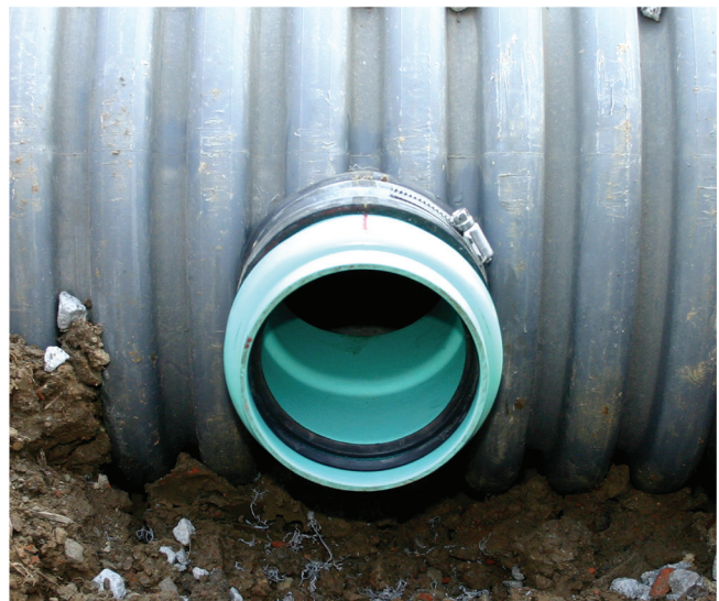
Inserta Tee Lateral Connection
