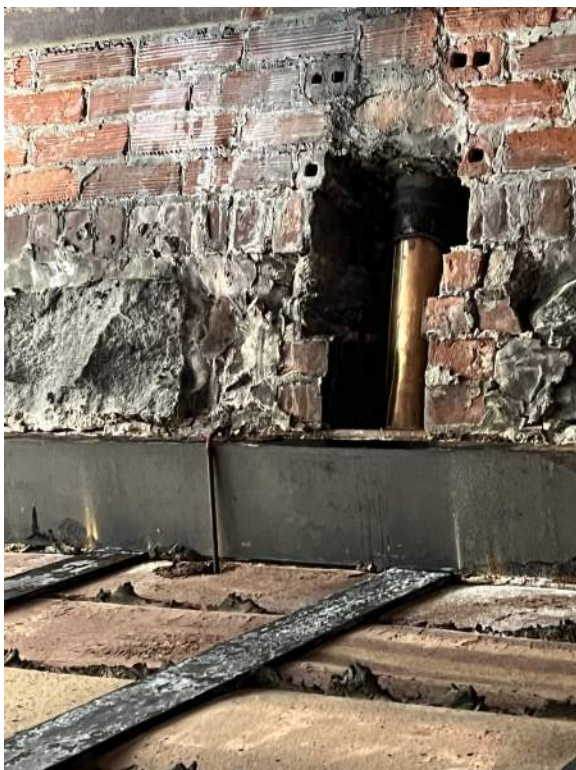
PHOTO 20 *NOT KEYED ON PLAN - INTERIOR VIEW OF ROOF DRAIN
