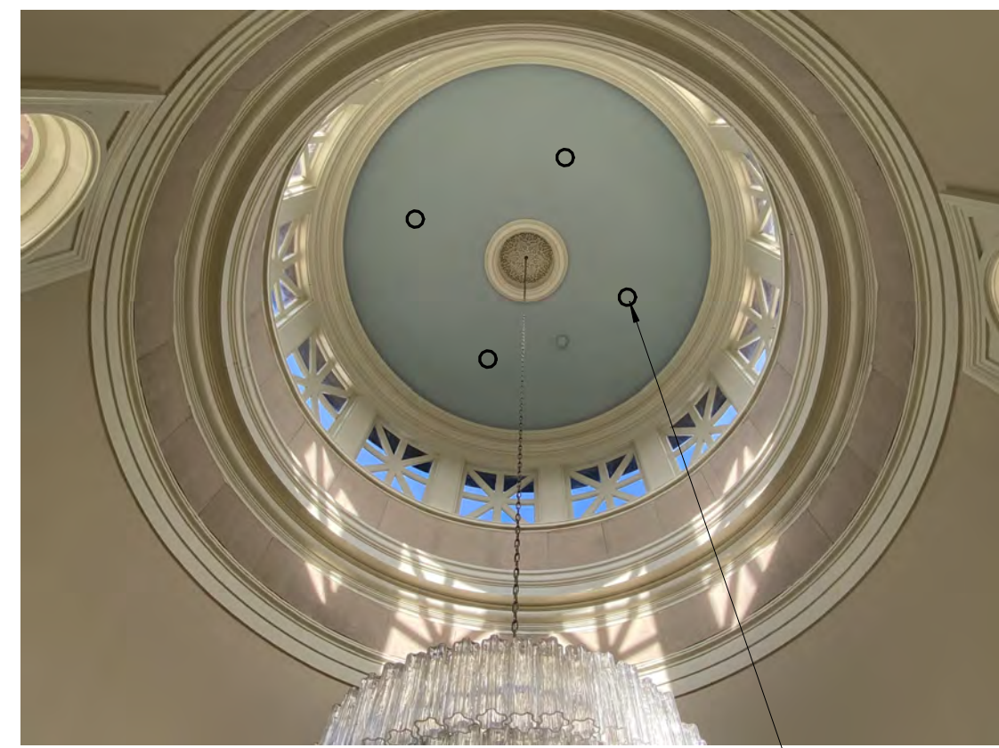
NEW SPRINKLER HEADS (TYP OF 4) AT DOME CEILING. COVERS TO BE FACTORY PAINTED TO MATCH ETR CEILING COORDINATE WITH FIRE PROTECTION DOCUMENTS AS REQUIRED.
